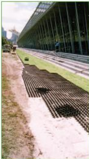
Melbourne Exhibition Centre during installation
