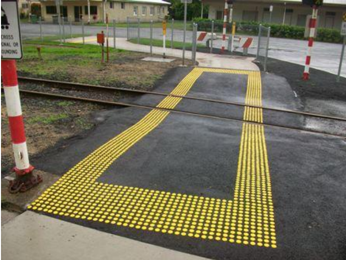
Yellow Polystud Installation – Babinda Railway Crossing
