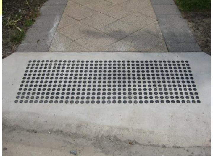
Black Polystud Installation – Cairns Port Redevelopment
