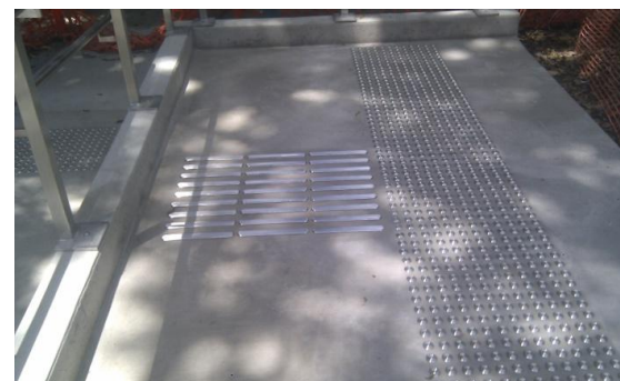
BELOW – Stainless Steel Indicators – Hazard and Directional Studs – Mossman Bus Stop
