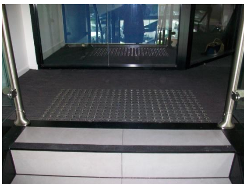
BELOW – Stainless Steel Indicators installed on carpet – Screw-In Type
