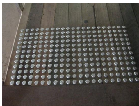
BELOW – Stainless Steel Indicators on timber surface – Cairns Port Redevelopment
